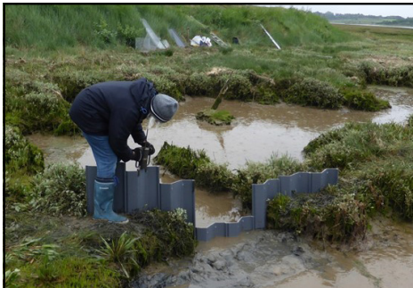
Positioning a sheet piling sill.
